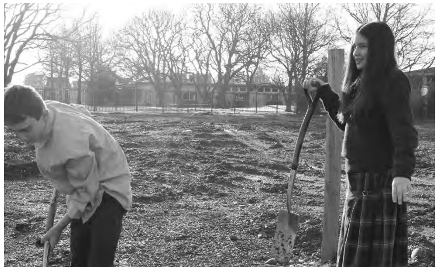
(Pictured above, left and right): College's two youngest students, Logan Bradford and Lilly Allen, undertaking the first turning of the earth on the site which was about to begin humming to the tune of machinery and building.
